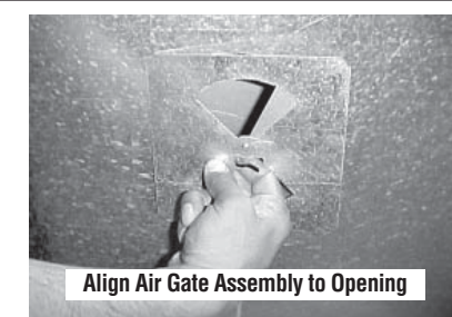
Figure 12 - Position Air Gate
