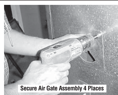
Figure 13 - Install Screws
