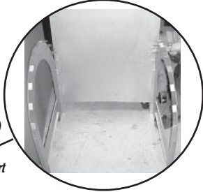
Figure 5 - Install Remaining Arch Support
